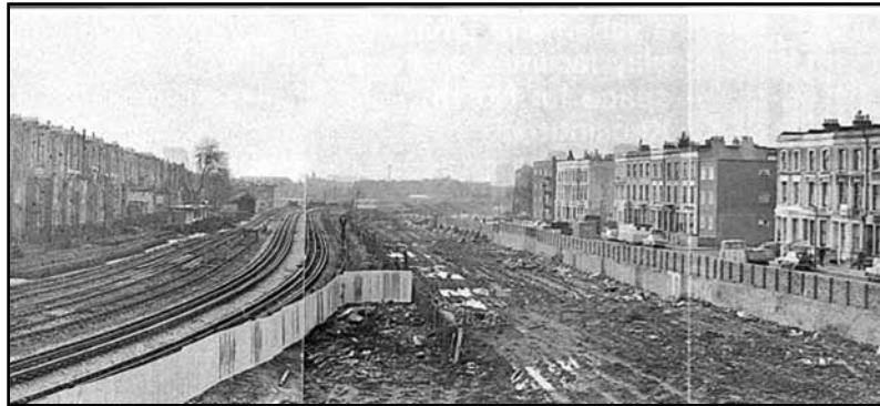
Western Ave. Construction, North Kensington, 1966
